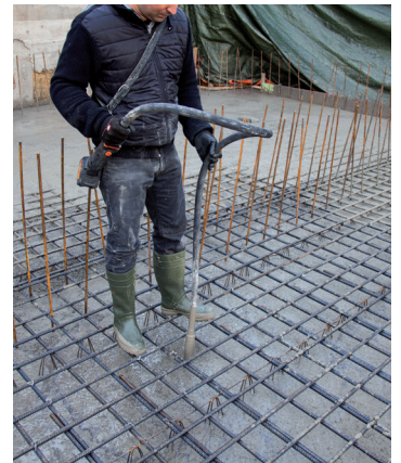
Effective compaction of concrete foundations
